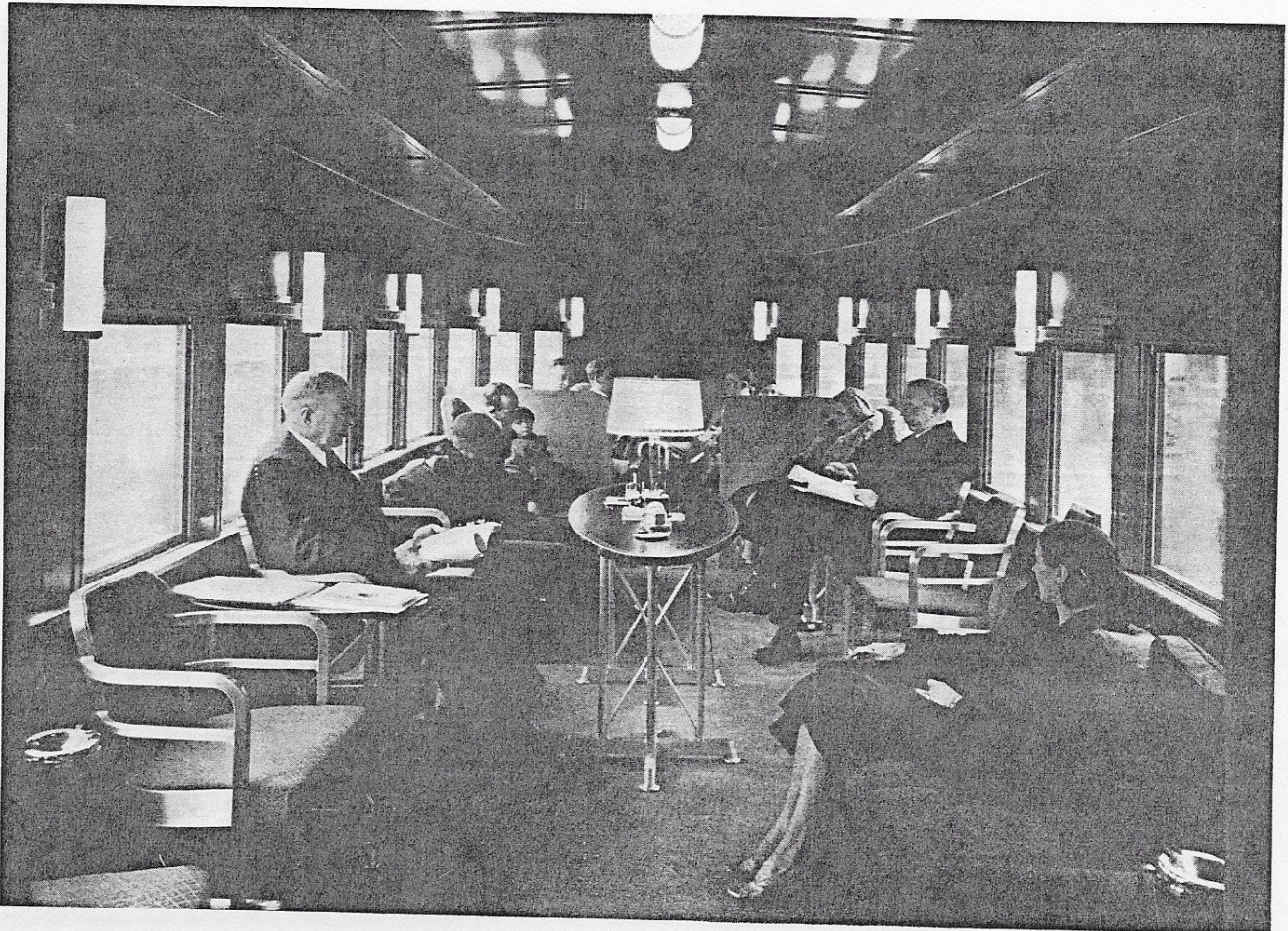
Club lounge or standard coach seats as specified. Double windows of safety and plate glass are fixed. Autotram is air conditioned, temperature automatically controlled. Lighting is modern and liberal.
